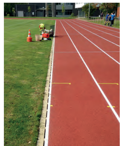
Slot channel: can be layered over on both sides
