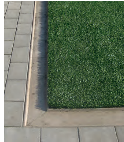
Trough channel for filled-pile artificial turf
