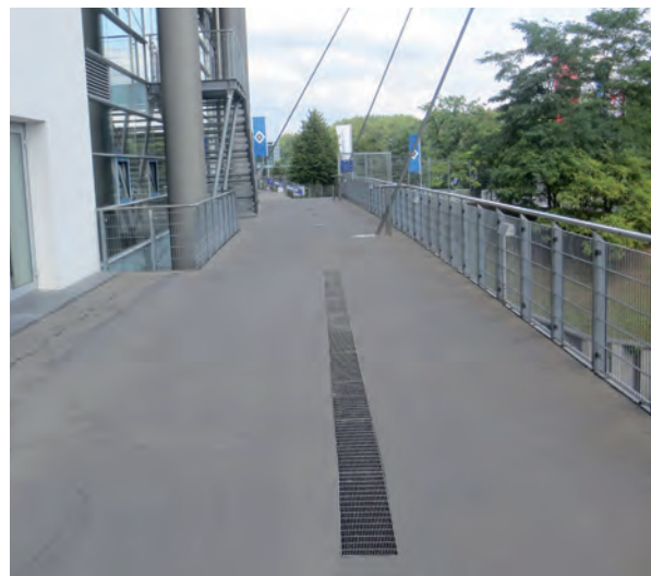
Stainless-steel channels for covered areas
