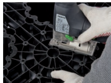
A keyhole saw with extra-long saw blade is required to cut out the openings for the pipe penetrations in the side panels and at the top of the basic elements
