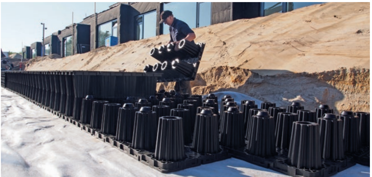
The system is constructed of basic elements that are laid in interlocking patterns
