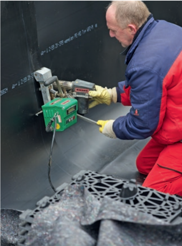
The sealing membrane is then welded
