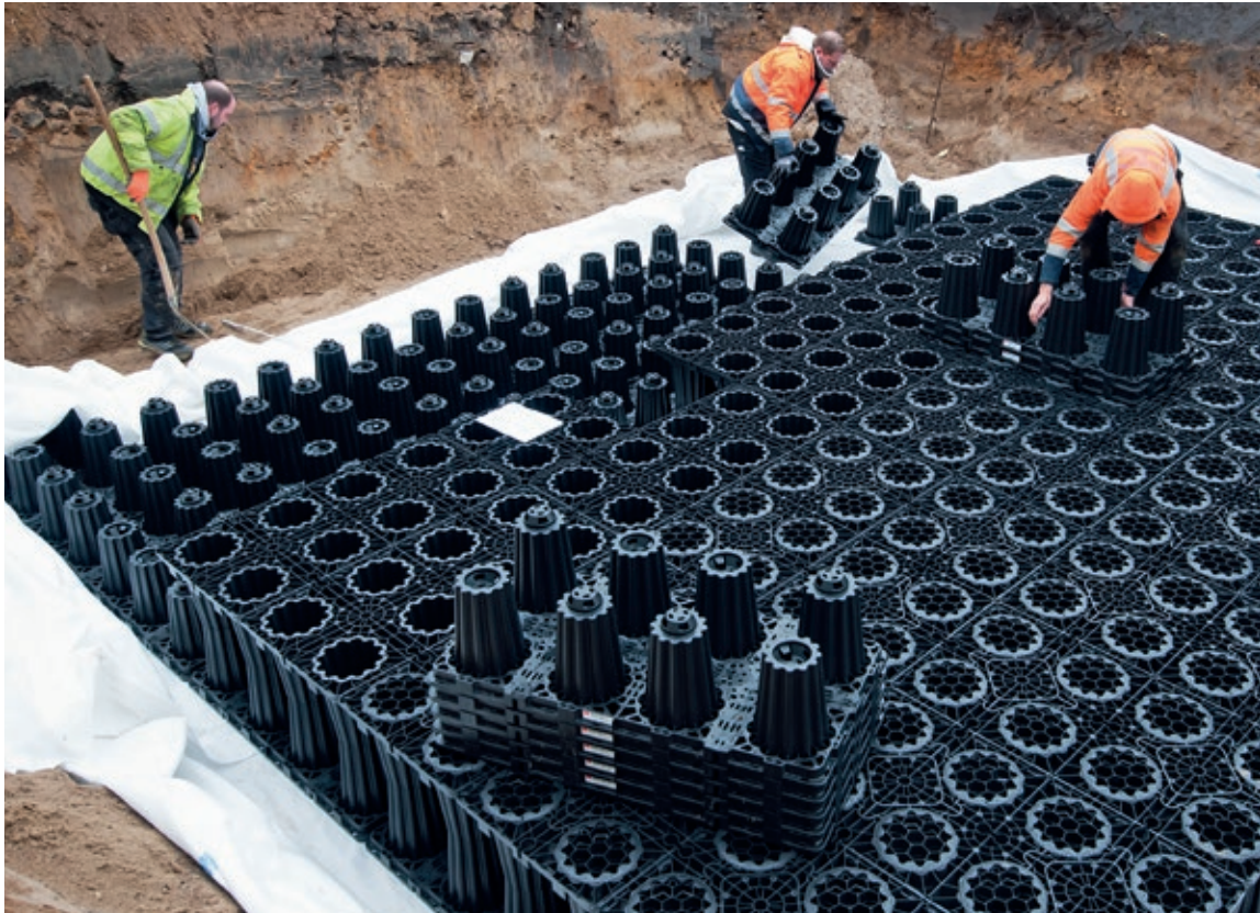
ACO Application Technology creates a corresponding installation plan for every building project. Reference project: Heider Marktpassage, Heide: ACO Stormbrixx HD as an infiltration system underneath car parking areas.
