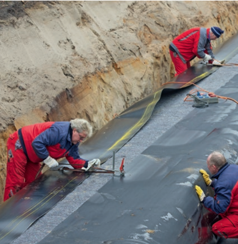
The bulk storage system is wrapped with an inner protective fleece and a sealing membrane
