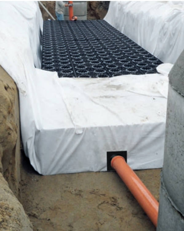
The protective geotextile is then laid around the infiltration system so that it is completely covered
