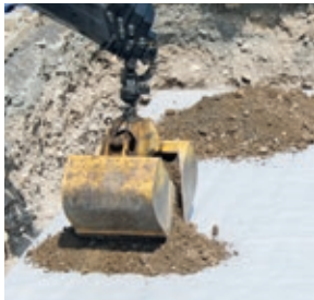
Filling the infiltration system
