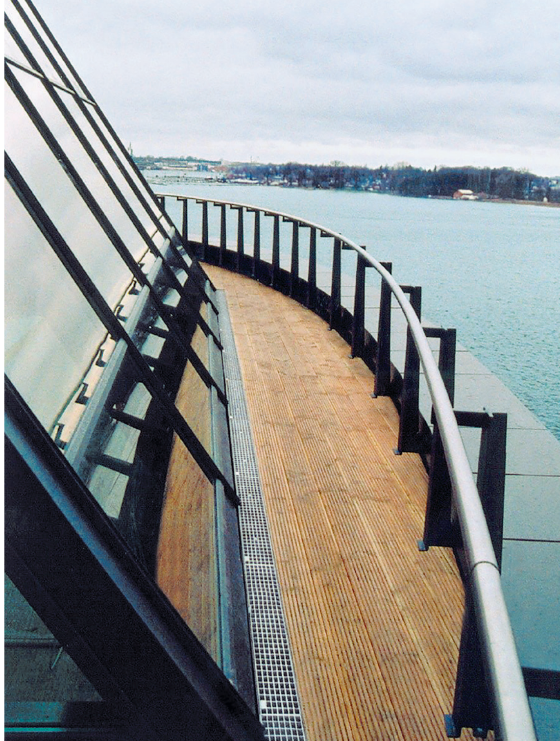
SIL04 Rostock, Germany ■ FACADE DRAINAGE
