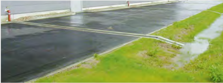
Drainage channels close to the surface discharge precipitation and rainwater quickly and easily into the infiltration troughs.
