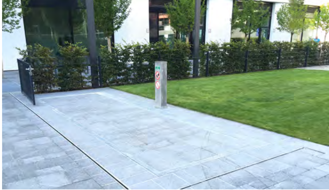
Special shaft covers offer the possibility of visual integration into the overall appearance
