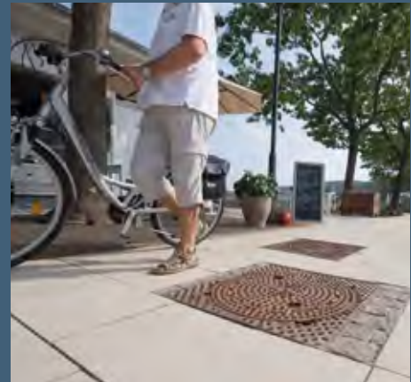
Square manhole covers blend in with the concrete blocks
