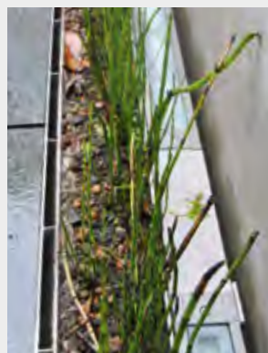
Accumulating rainwater is collected and routed to a trough near the surface
