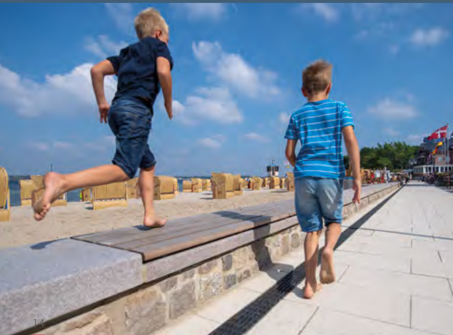
New sand-coloured concrete pavement, natural stone wall, benches and drainage
