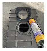
7 Once the outlet has been cut away, place a bead of our recommended sealants, such as Sikaflex 11FC or Geocel 945 into the sealant groove on the outlet connector.
