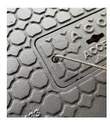
4 Once you have lubricated both of the locations, the access cover should be placed back into position and fixed down.
