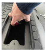
Working on the right-hand access channel facing the road, take your lithium white grease can and spray down the expansion joint through the opening on top of the channel.
