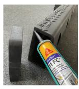
Once cut, install the end cap using a recommended sealant such as Sikaflex 11FC or Geocel 945.
