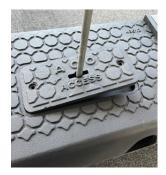
1 Untighten and then remove the access covers located on the top of the access channels at either end of the expansion joint.
