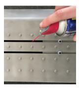
When the slots on the cover are open, you should also spray white lithium grease through these slots onto the top of the moulded expansion joint below.
