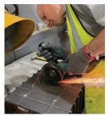
3 Using an angle grinder with a 1mm disc attached, cut through the base of the channel separating it into four segments (see example above).
