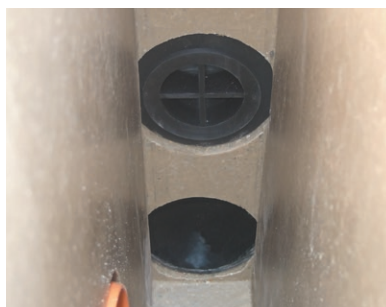
View of foul air trap before installation
