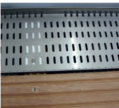
The channel body is screwed into the channel base through the 4 mm drainage slot
