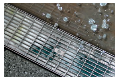
Water level up to the lower edge of the cover grating
