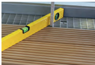
Fitting of the wood terrace channel
