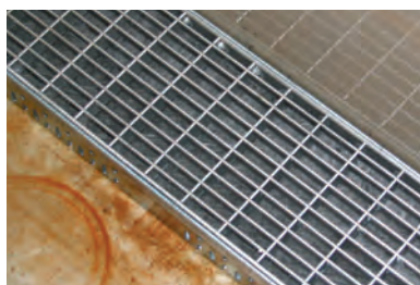
When clean, an inserted dirt fleece reduces the hydraulic performance of the system by 30%
