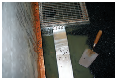
Test set-up with branch channel lateral (without a section in the gully top for roof gullies)
