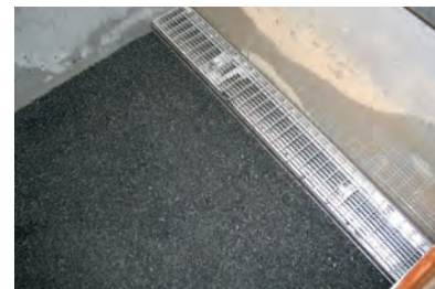
Gravel bed with 2/5 mm gravel
