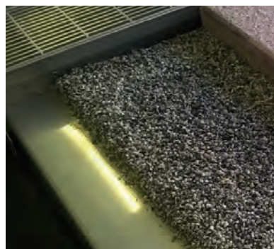
Inserting the gavel and installation the block pavement
