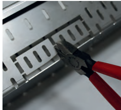
Opening the branch channel connection
