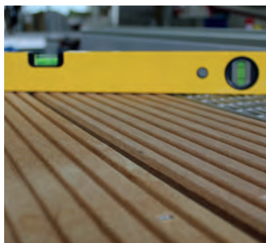
Check the installation height
