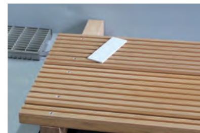
If necessary, place material below the channel body
